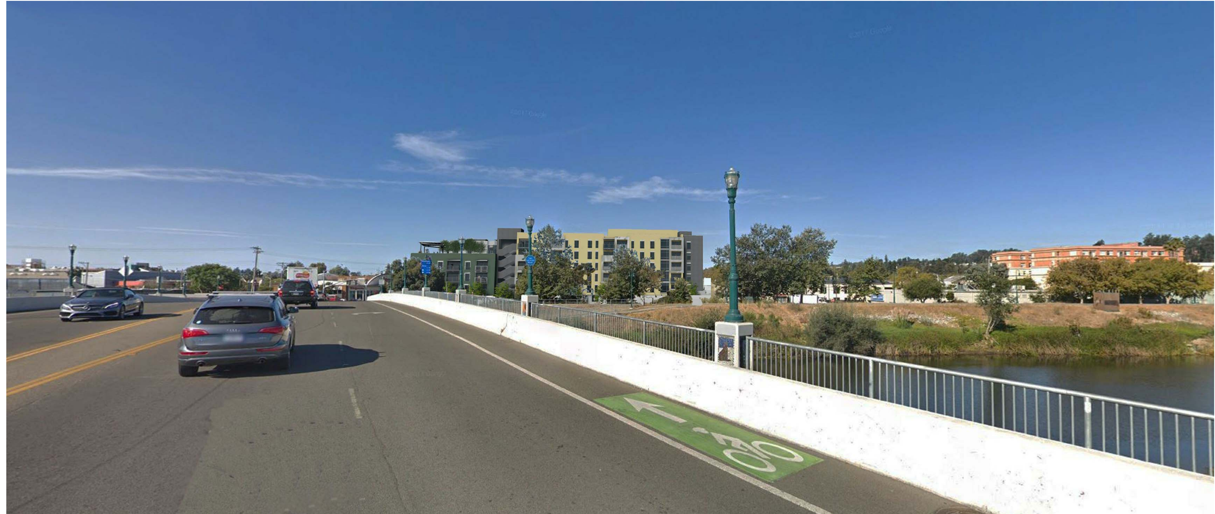
5 VIEW FROM ACROSS LAUREL STREET BRIDGE
