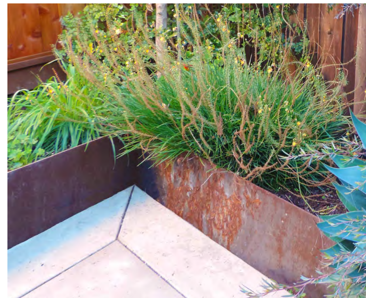
RAISED CORTEN STEEL PLANTER (PHOTO BY JLJA)
