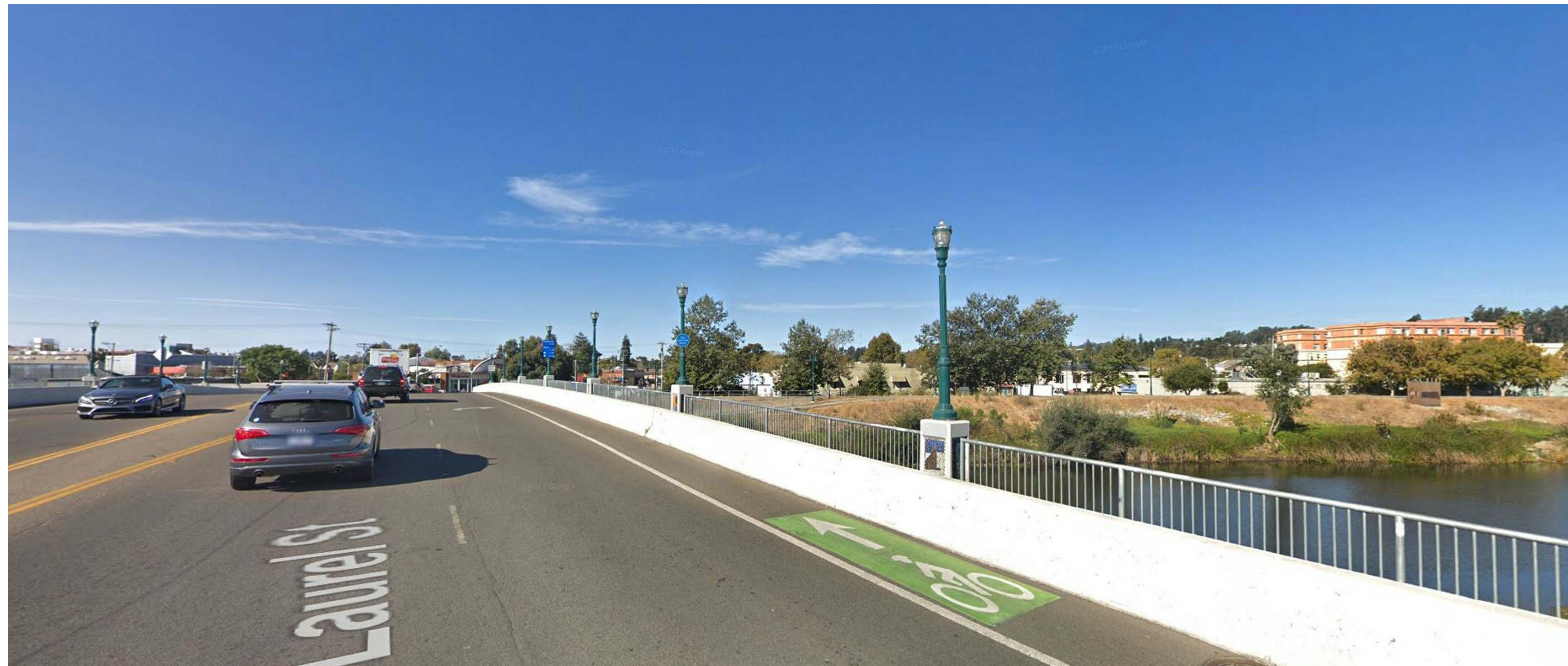
5 VIEW FROM ACROSS LAUREL STREET BRIDGE
